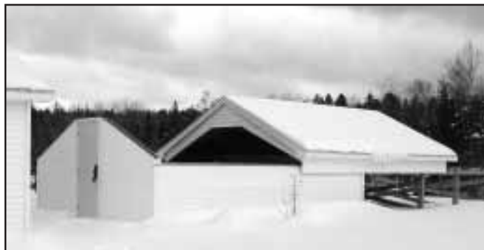
The roll-off with the roof partially open.
