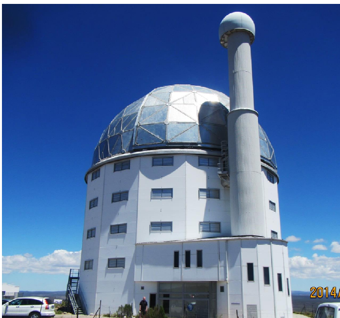
A view of the telescope building, dome and alignment tower
