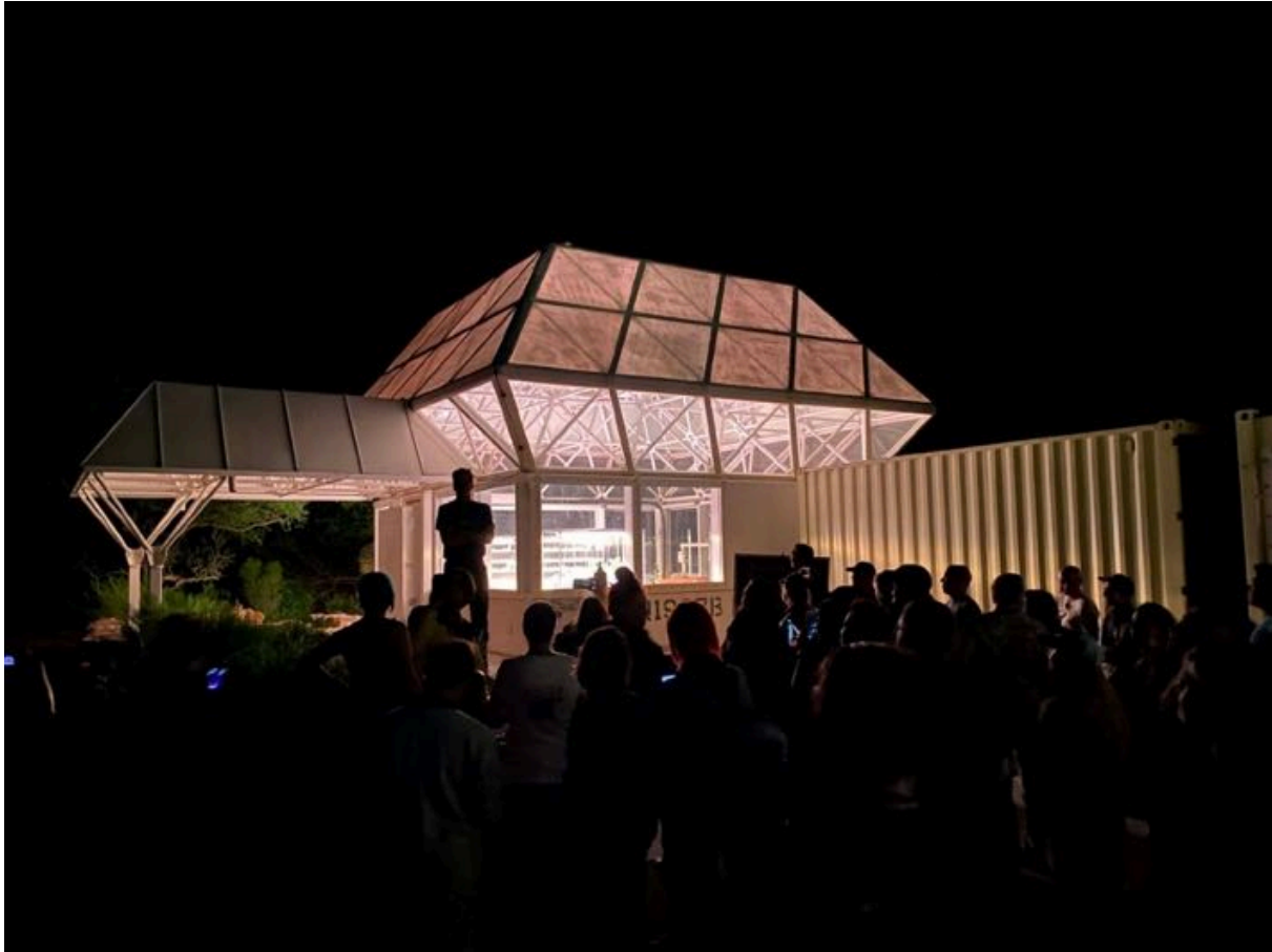
Mars/Moon Analog habitat (under construction)
